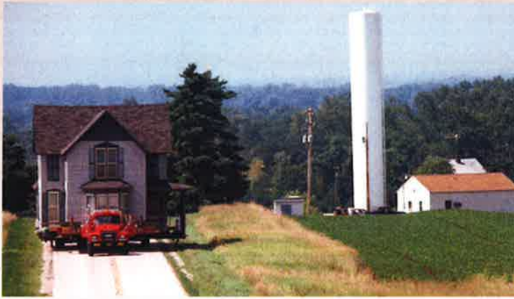
Moving of 2 homes to the new town site.
