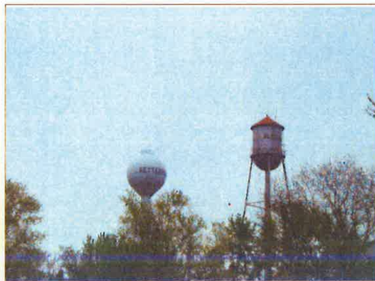
Keytesville Water Towers (Old and New)—2007
