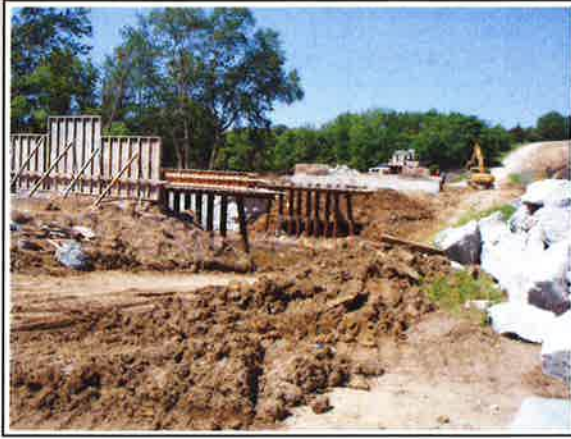
Mercer County Bridge in Progress
