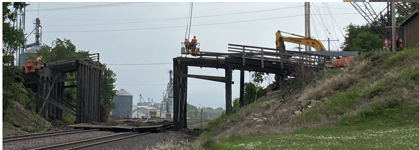
Trenton 17th Street Bridge Project
