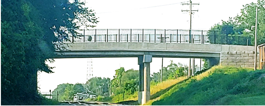
17th St. Bridge Project, Trenton
